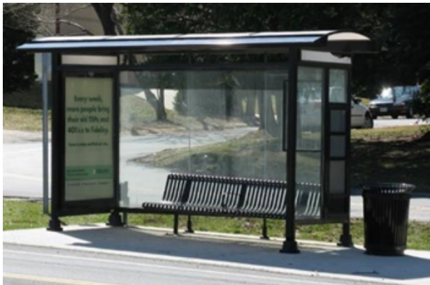
Figure 75. Example of bus shelter Source: volokh.com
