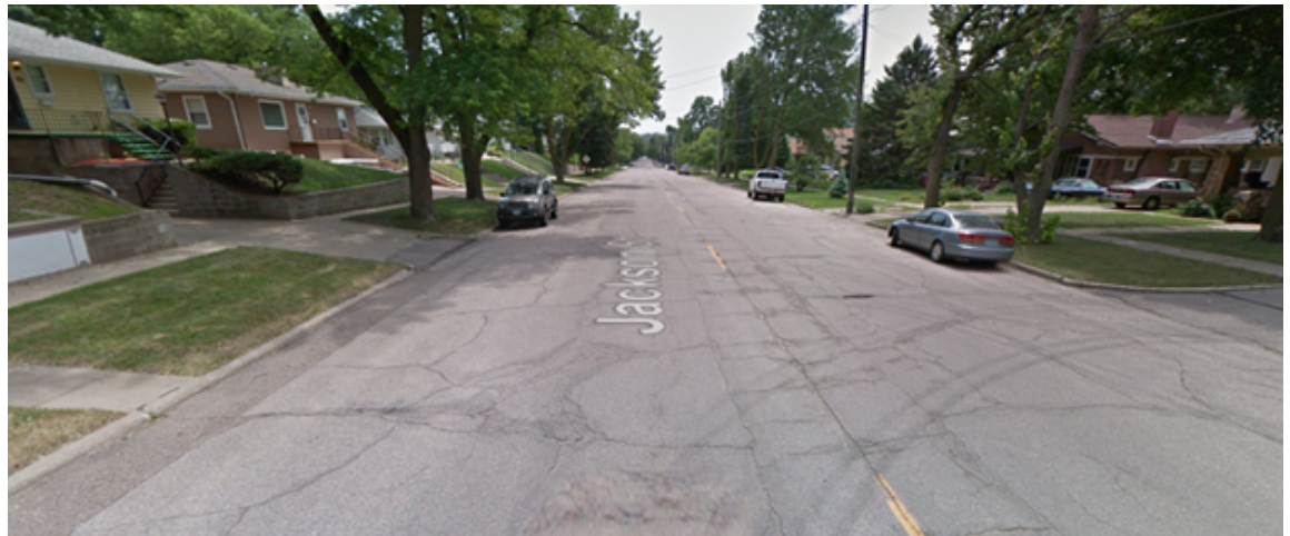
Figure 40. Jackson Street: Existing conditions
