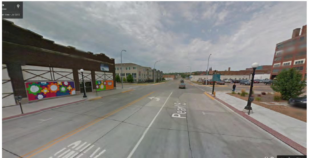
Figure 36. Pearl St.: Existing conditions
