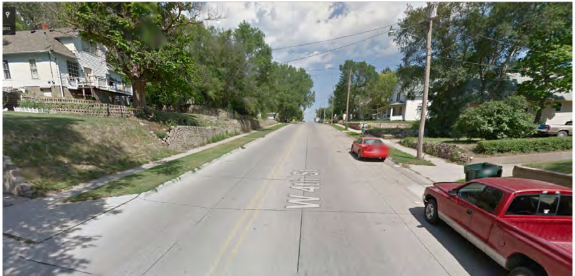
Figure 56. West 4th St.: Existing Condition
